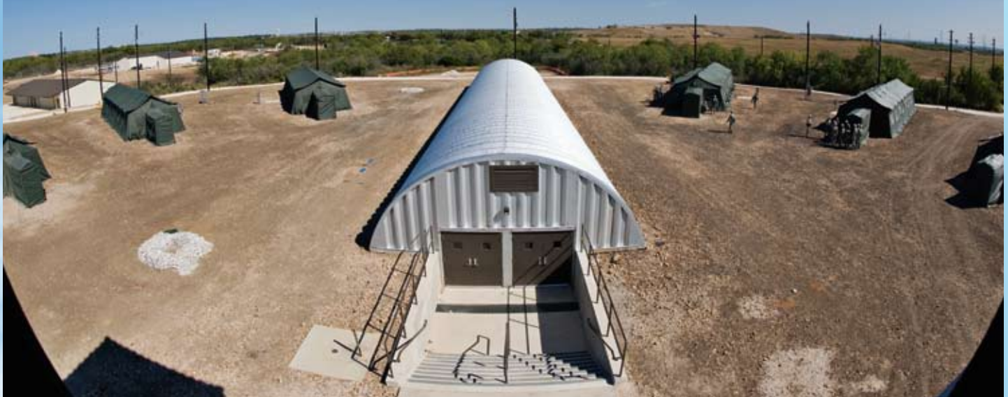
The Basic Expeditionary Airman Skills Training course, or the BEAST, is a new facility added for the two additional weeks of basic military training and replaces “Warrior Week.” The $28 million course consists of four zones, called tent cities. Each zone, designed to immerse Airmen in realistic training, consists of 10 tents, one latrine, one hard shelter and one tower.
