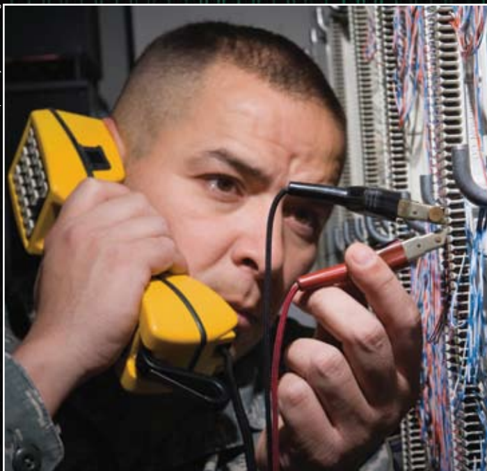
Telecommunications specialist Master Sgt. Johnnie Hernandez taps into a PBX distribution panel to check a phone line at the Defense Media Activity - San Antonio. The Air Force Information Operations Center executes a comprehensive program to help protect Air Force telecommunications switch systems and services. An important component of this program is a capability to monitor transmissions to identify unauthorized dial-up modems, suspect telephone call patterns and other unusual activities.
